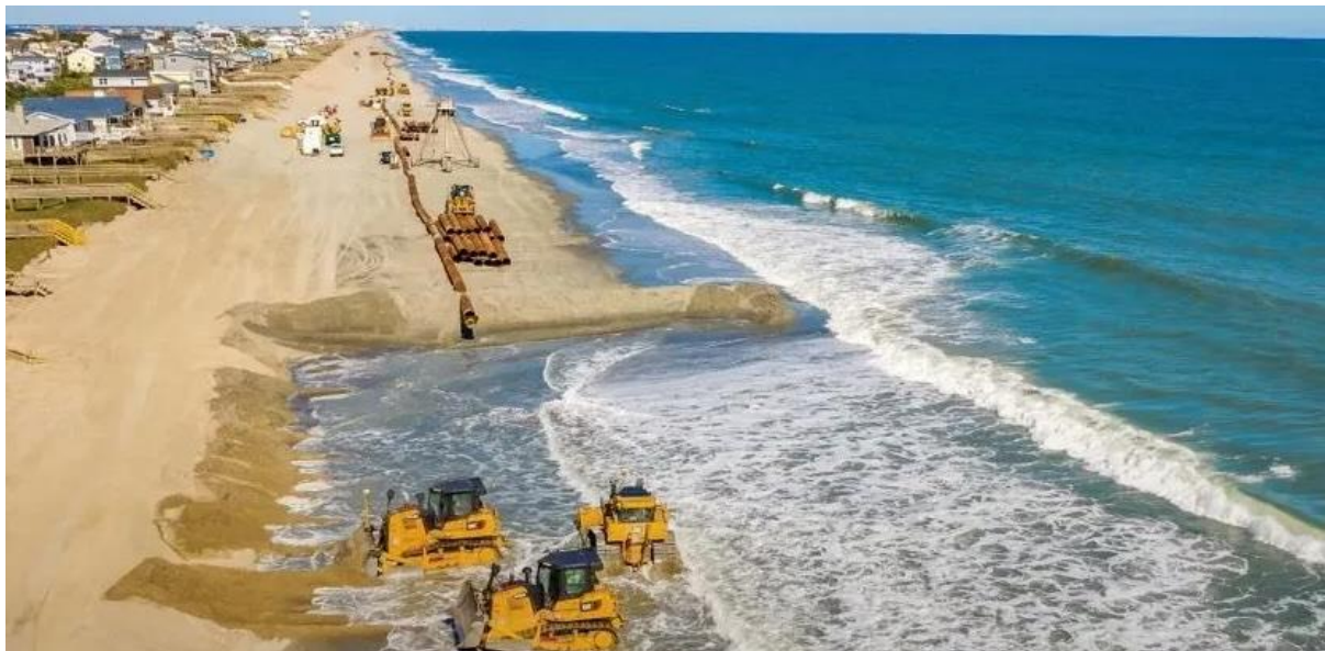
Figure 1. Beach face nourishment at New Jersey Shores, United States. Credit: GLDD.
