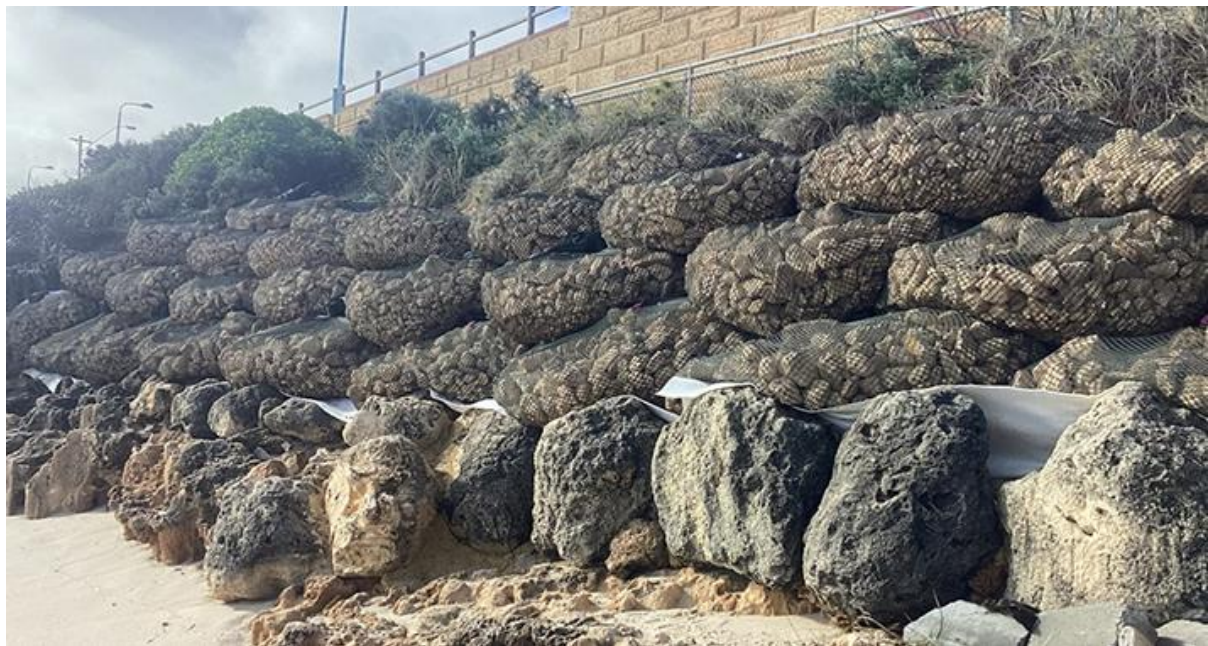
Figure 31. Rock filter units for coastal erosion control in the City of Sterling Credit: City of Stirling.
