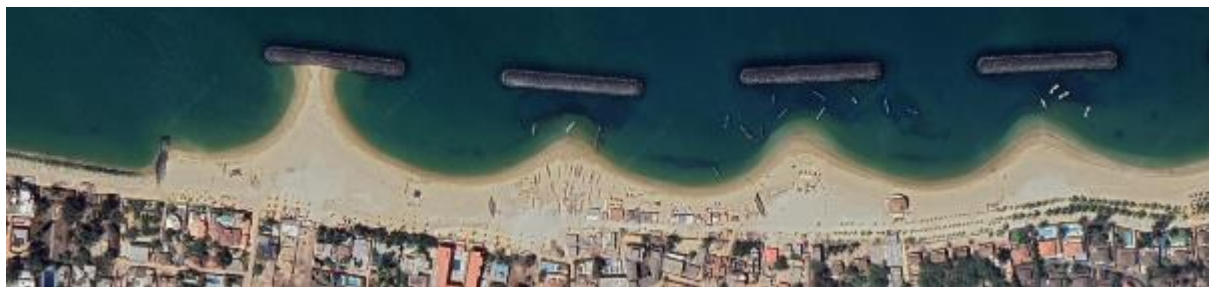
Figure 16. Detached breakwaters at Saly Beach, Senegal. Credit: Google Earth.
