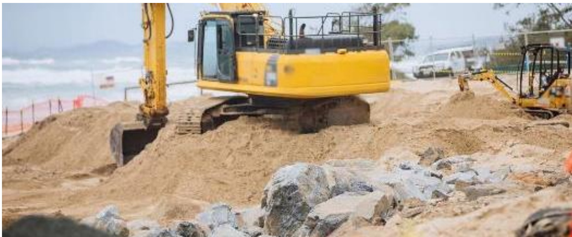
Figure 19. Hybrid seawall-dune system construction on the Gold Coast, Queensland: a seawall core buried beneath sand, then capped with additional sand and stabilised through dune revegetation. Credit: ICM.
