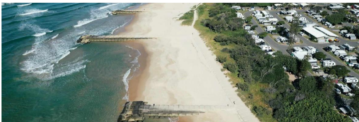
Figure 11. Geofabric groynes at Maroochydore, Australia. Credit: ICM.
