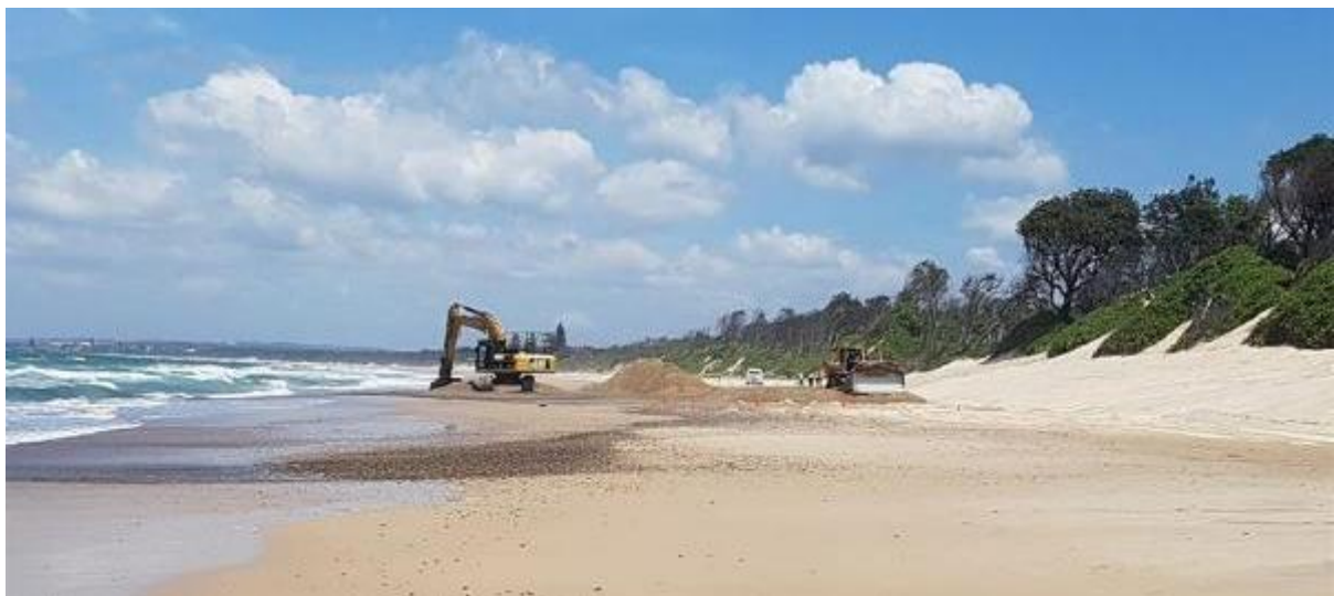
Figure 5. Beach scraping at Old Bar Beach, NSW. Credit: Coastal Wiki.
