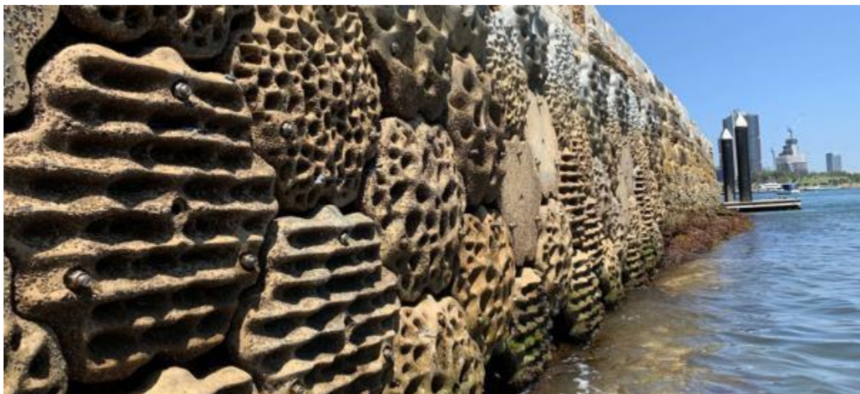
Figure 30. Living Seawalls in Sydney, NSW. Credit: Adapt NSW.
