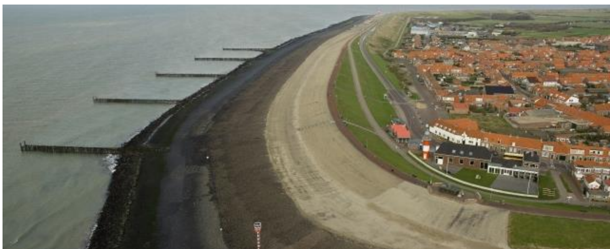
Figure 15. Sea dike in the Netherlands, combined with longshore control structure. Credit: Coastal Wiki.
