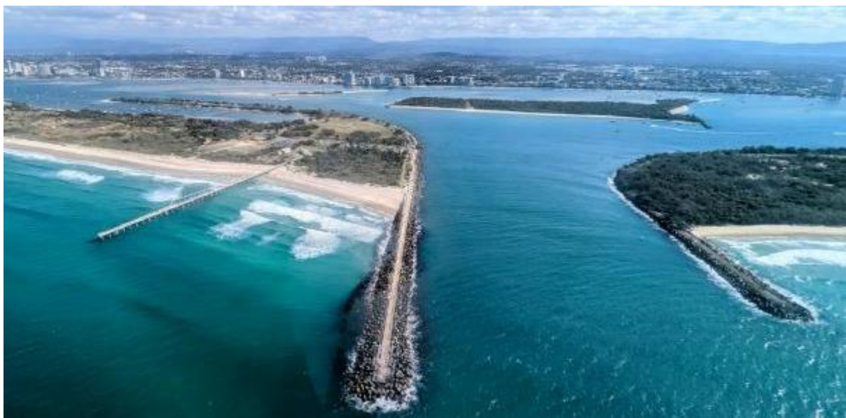
Figure 3. Tweed River Sand Bypass System. The Jetty captures the sand which is transported north across a series of pipes underneath the river. Credit: Gold Coast Waterways Authority.
