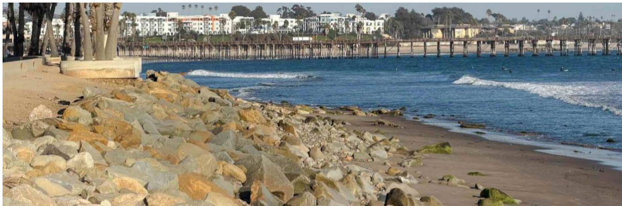
Figure 20. Dynamic cobble berm at Surfer's Point, Ventura, California. Credit: ICM.
