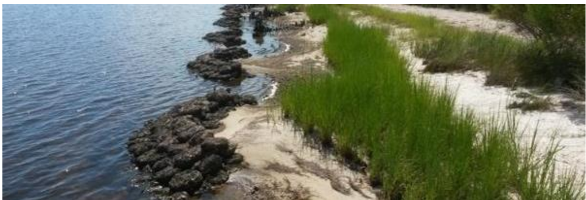
Figure 29. A Living Shoreline constructed in Panama City, Florida using plants and oyster shell. Credit: Florida Living Shorelines.
